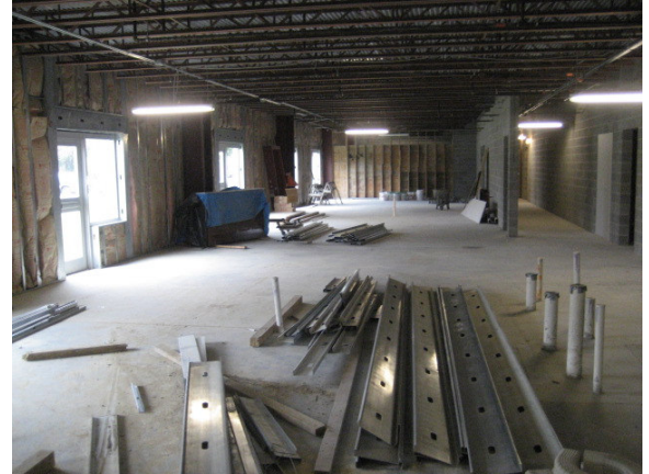
Preschool area under construction
