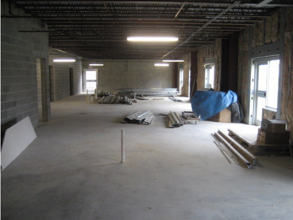
Preschool area under construction
