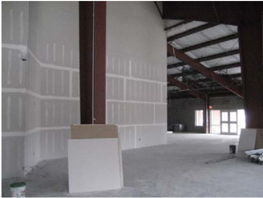
Game room under construction
