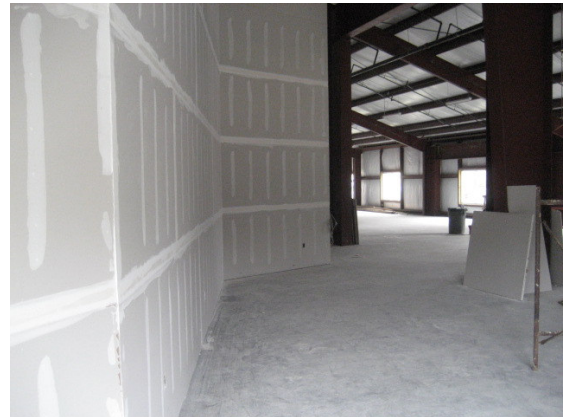
Weight room under construction
