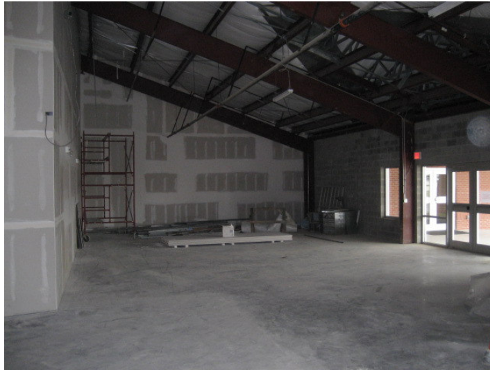
Parlor under construction
