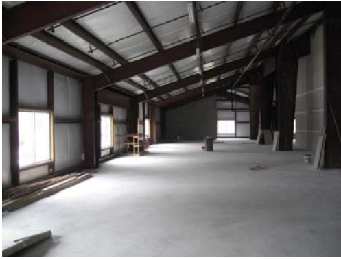
Adult classrooms under construction
