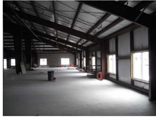
Adult classrooms under construction
